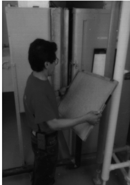
Replacing filters regularly is an easy way to get high air quality, low energy use, and long life for your heating and cooling equipment.
