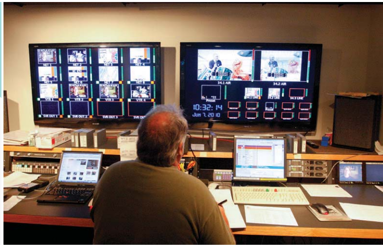
(Left) A control room at the new WNIT building. (Below) The studio in the new WNIT building boasts the largest studio in the state.
